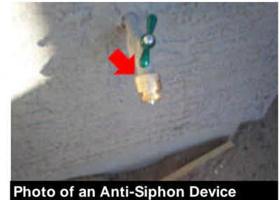
Photo of an Anti-Siphon Device
